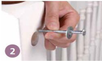
2 Unscrew and remove the bolt holding the handrail and keep safely.
