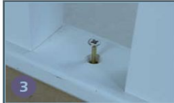
3 Unscrew the floor rail.
