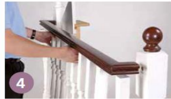
4 Once all the fittings have been removed, the section of assembled balustrade is simply lifted off.
